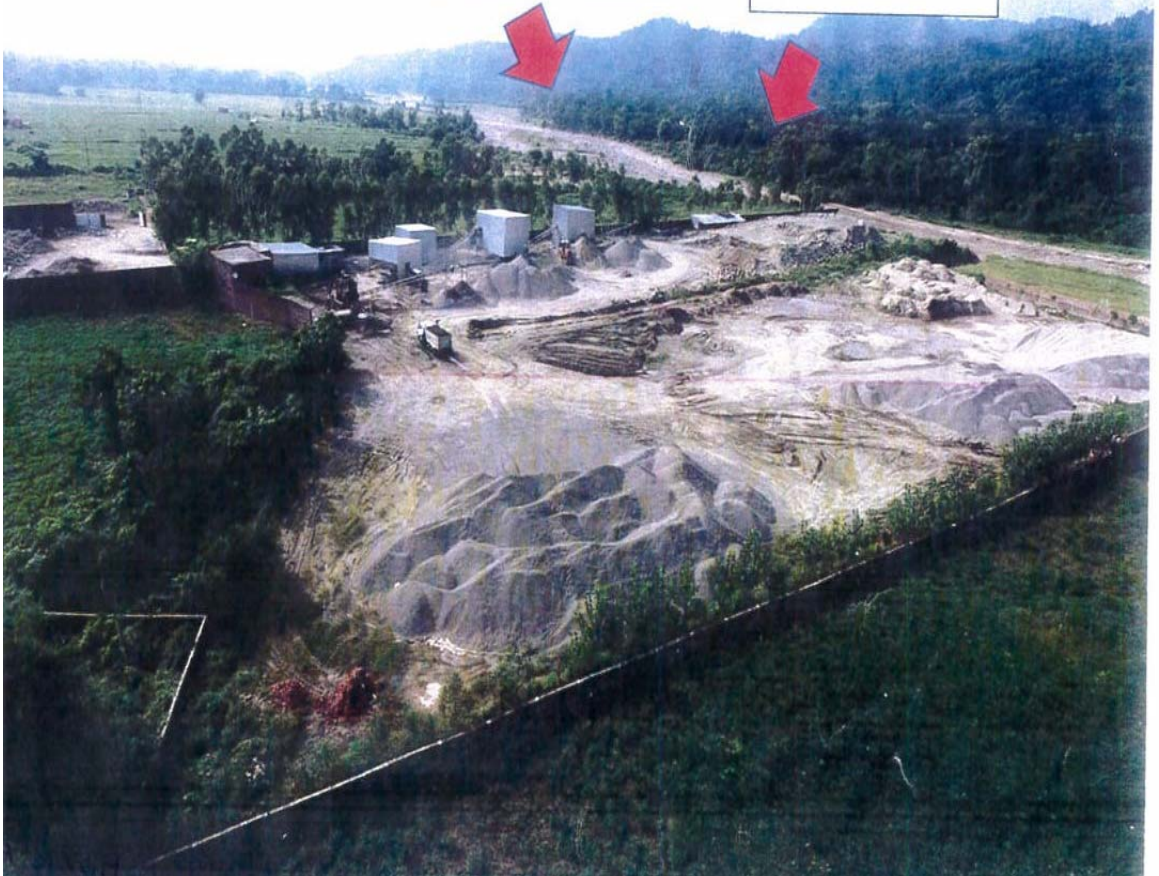
Waste water Outlet
