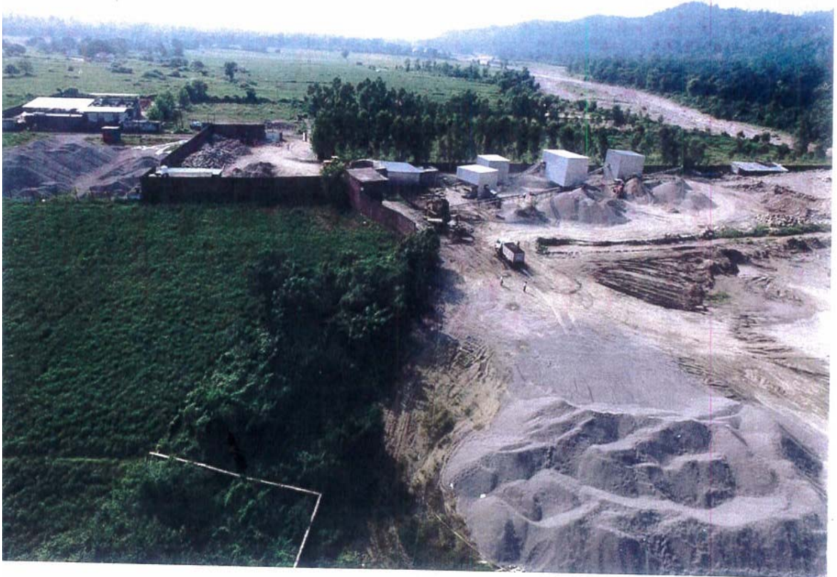
Illegal excavation & its loading and unloading
